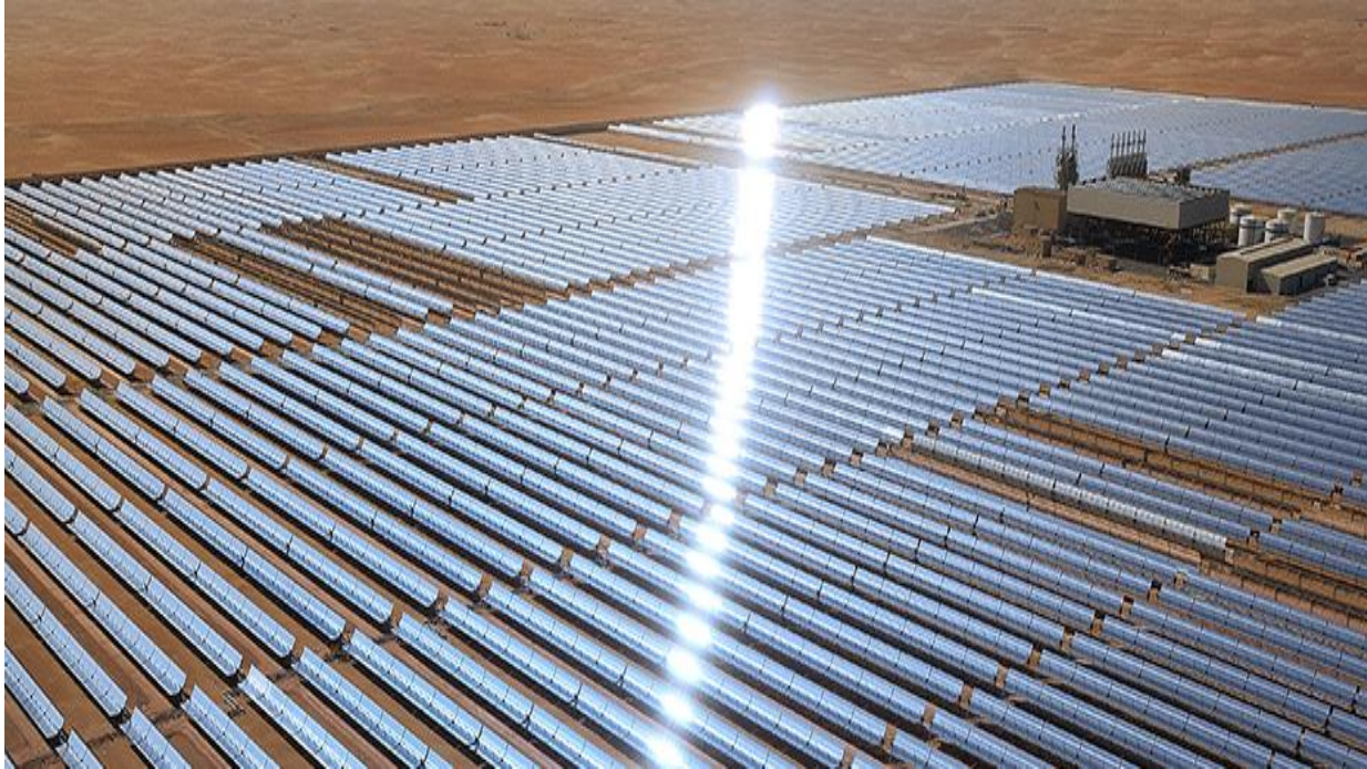
Shams Plant in Zayed City, UAE
