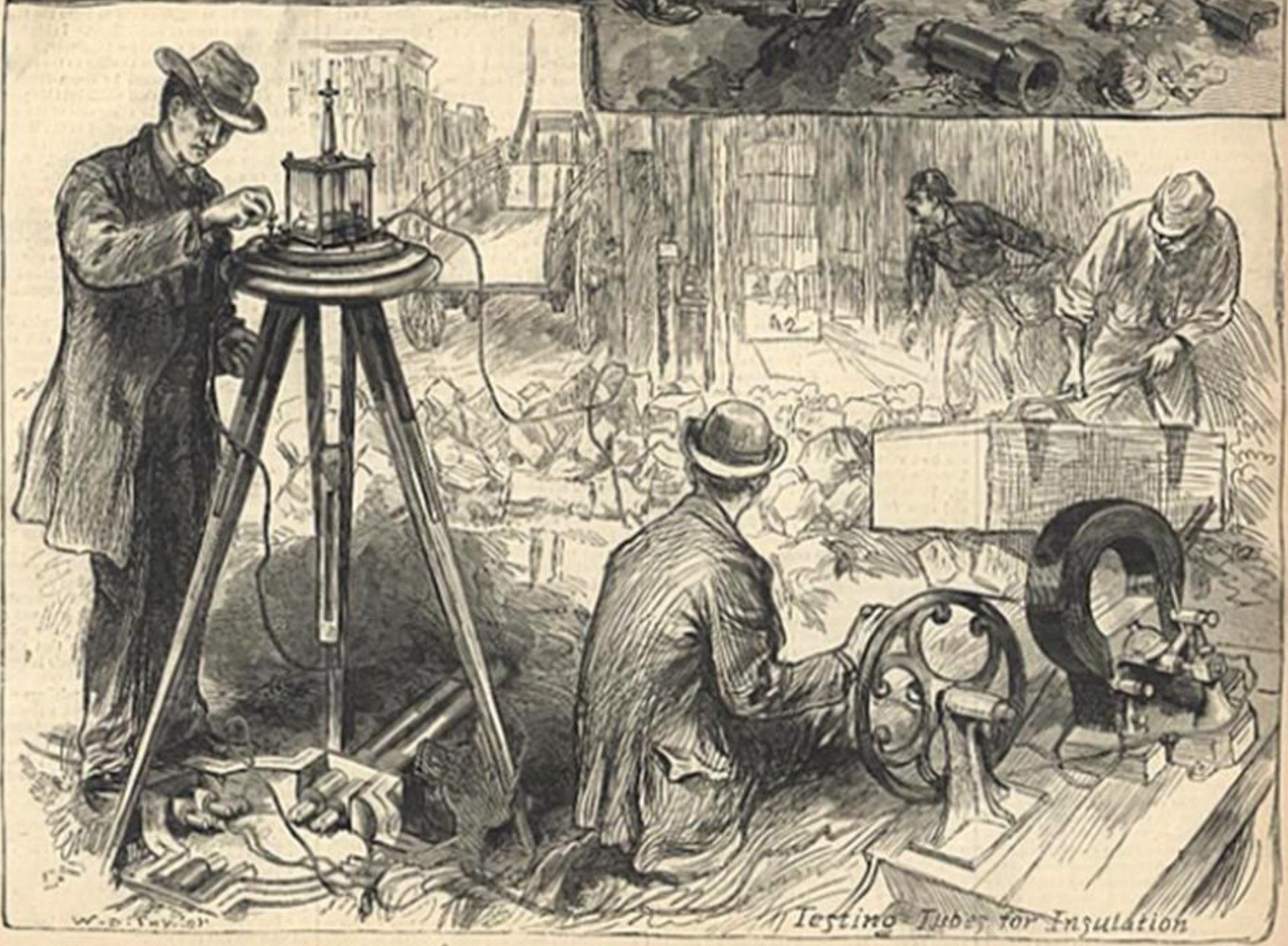
Laying the Electrical Tubes
