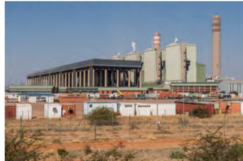
A general view of Medupi Power Station completed on 5 August 2021 in Lephalale, South Africa. Picture: Gallo Images/Rapport/Deon Raath
