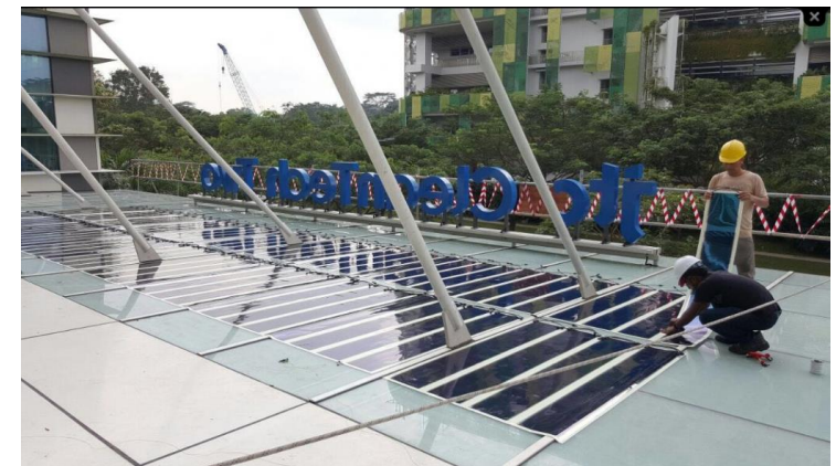
Singapore Cleantech Building Façade with HeliFilm installation
